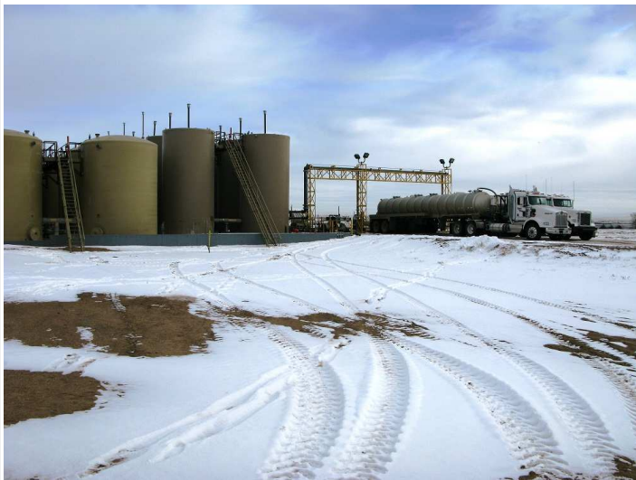
Oilfield waste arrives by tanker truck at a wastewater disposal facility near Platteville, Colo. After removal of solids and oil, the wastewater is injected into a deep well for permanent storage underground. This disposal process has the potential to trigger earthquakes, but very few wastewater disposal wells produce earthquakes. No earthquakes are associated with injection at the site in this photograph. Photo taken on Jan. 15, 2013. Photo Credit: William Elsworth, USGS
