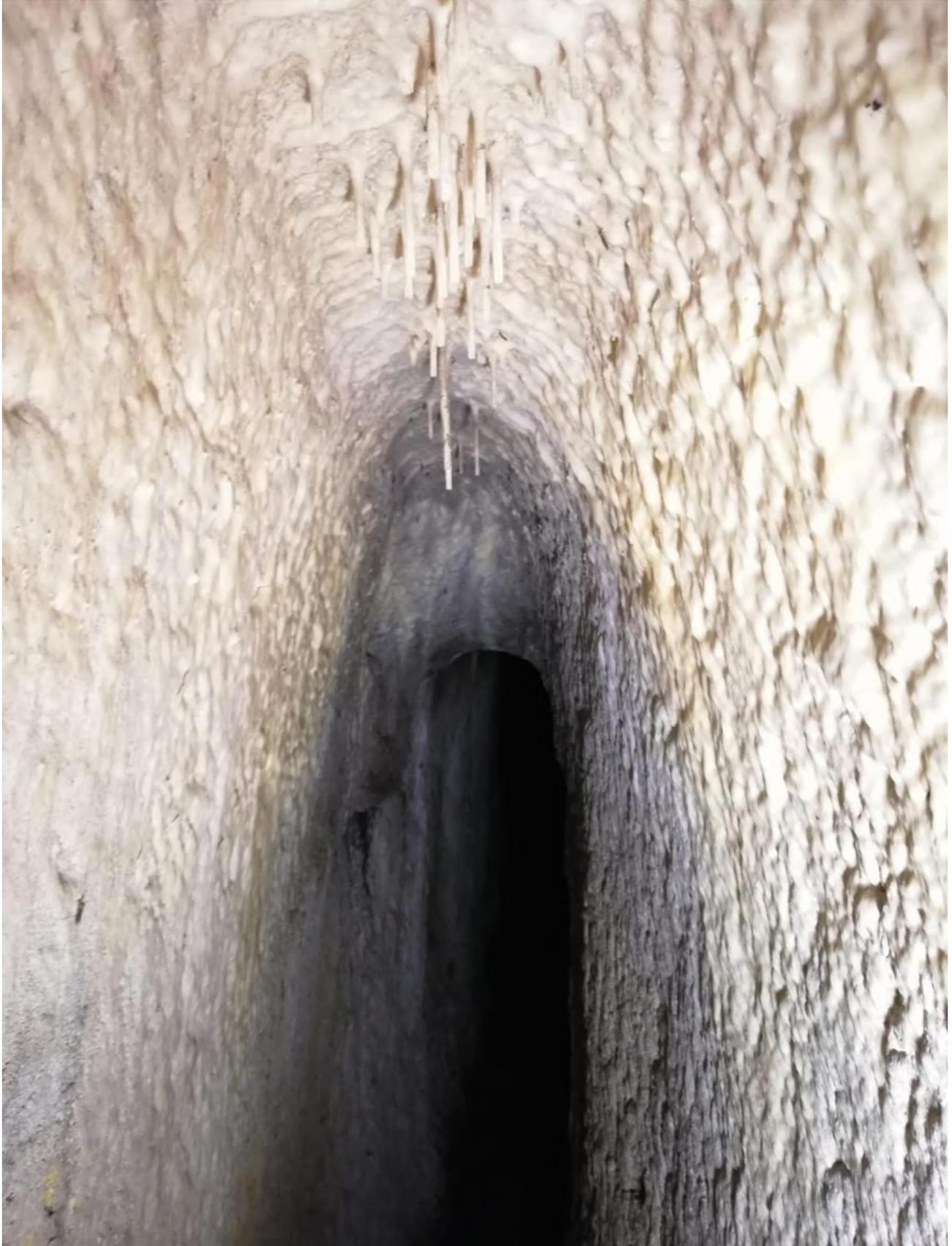
**Fig. 21** – Presence of calcium carbonate statallites inside the ancient tunnel explored on 9 September 2021. Giancarlo Valle, Credits: Arco di Diana APS.
