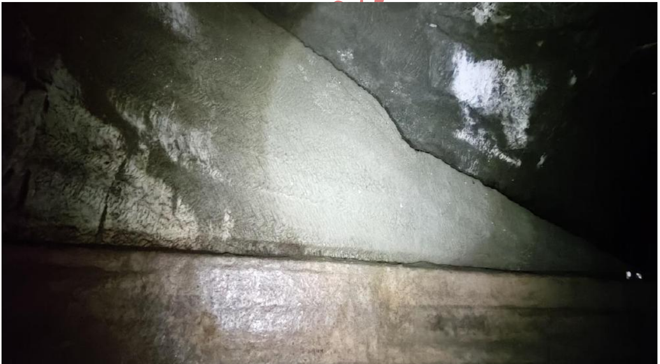
Fig. 10 - Hypogeal Area - North perimeter structure. A large concretion of calcium carbonate is observed. Credits: Daniele Cataldi, Riccardo Bellucci, Settimio Tersigni, Marco Tudini.
