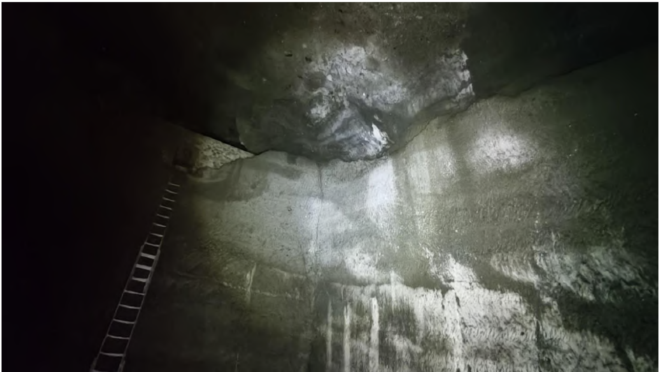
Fig. 9 - Hypogeal area - N, S perimeter structure and part of the ceiling. A large concretion of calcium carbonate is observed. Credits: Daniele Cataldi, Riccardo Bellucci, Settimio Tersigni, Marco Tudini.
